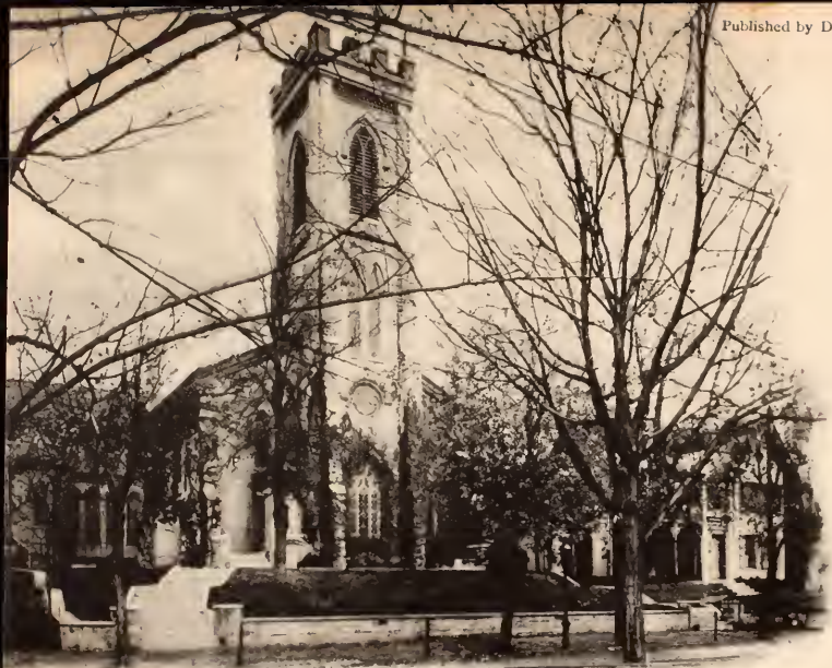
ST. JOHN'S EPISCOPAL CHURCH AND RECTORY, NORRISTOWN, PA.
